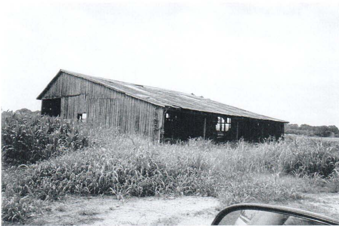
Figure 6 - Photograph of north machine shed (looking northwest)
