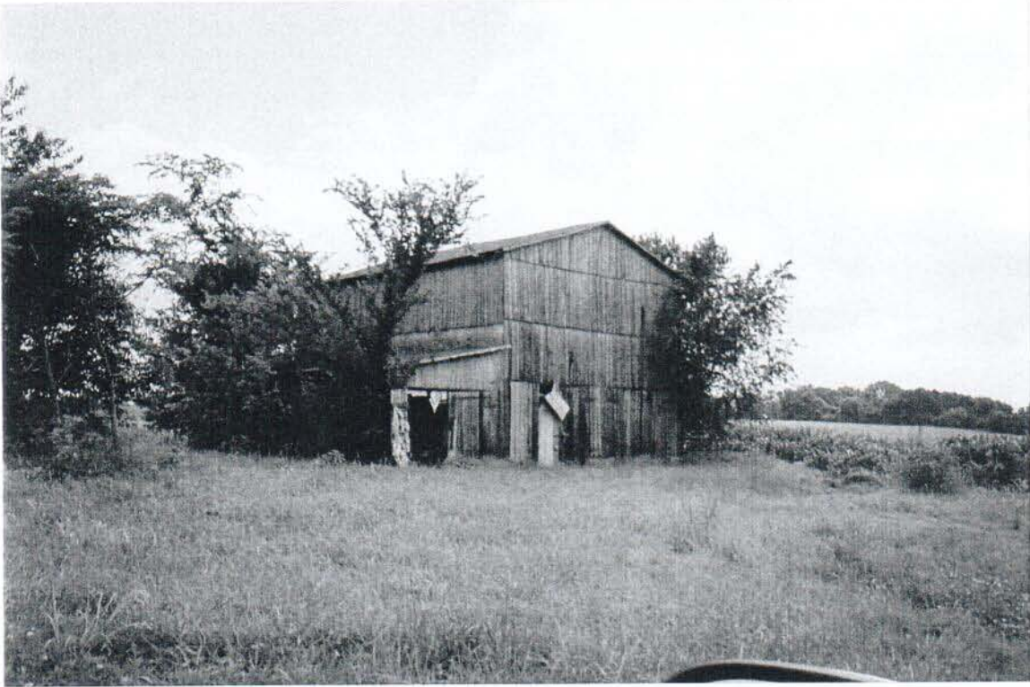
Figure 5 - Photograph of tobacco barn (looking southwest)
